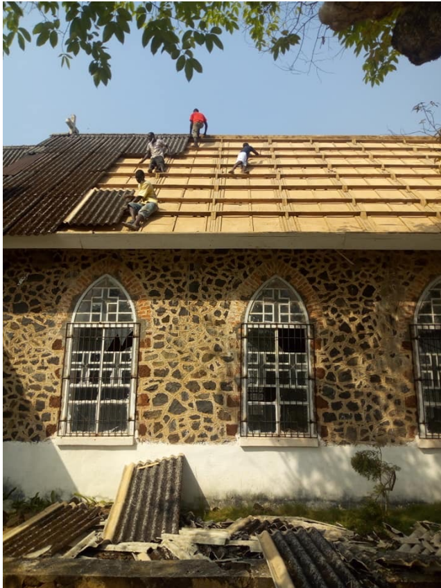
Roof with asbestos tiles
